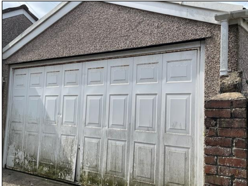
Figure 7 Photo of Rear Elevation of Property
