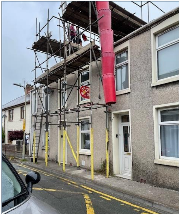
Figure 5– Photos of front elevation of property Photo (taken 13/06/2024) looking along St Marie Street. contractors were removing chimneys
